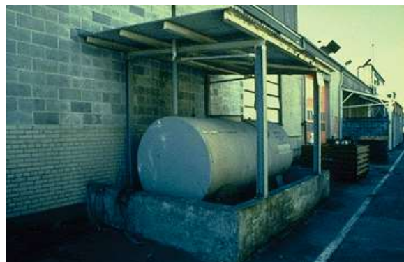
Covered AST with secondary containment
